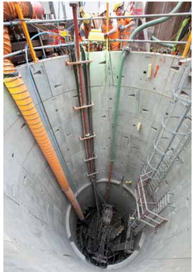
Uno de los pozos conocidos como ‘grout shaft’ que se excavará en las futuras estaciones de Bond Street y Tottenham Court Road. One of the shafts known as ‘grout shafts’ that will be excavated in the future Bond Street and Tottenham Court Road stations.
