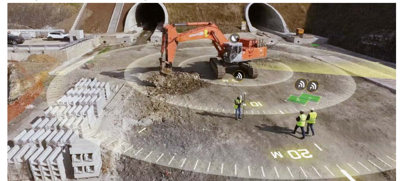
El sistema Warning Presence of People avisa del riesgo de atropello en las inmediaciones de maquinaria pesada. The "Warning Presence of People" system warns of the risk of being run over in the vicinity of heavy machinery.
